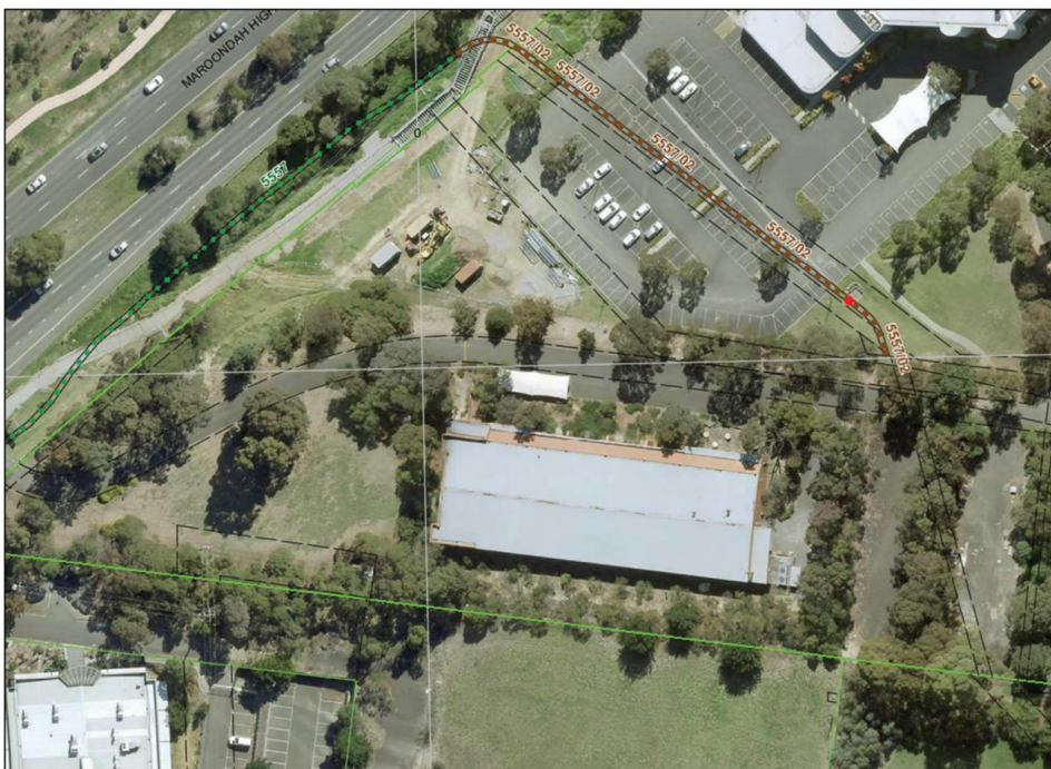
Figure 7. Melbourne Water main drain
